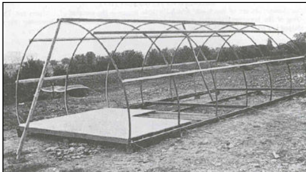
Wooden flooring is installed, the inner corrugated lining (horizontal) added, then the end piece and outer corrugated skin (vertical) applied. (Images from Nissens.co.uk)
